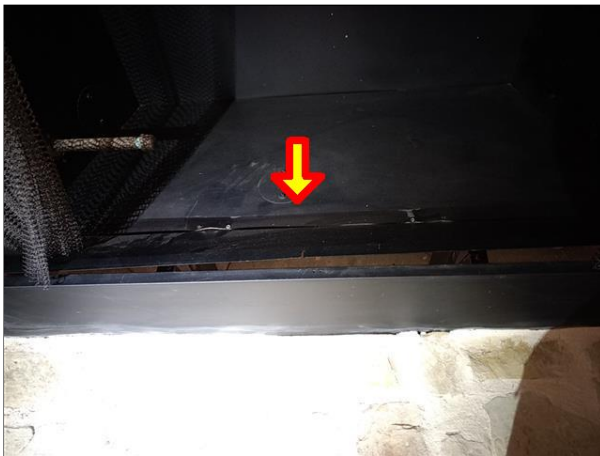
floor is thin gauge metal
