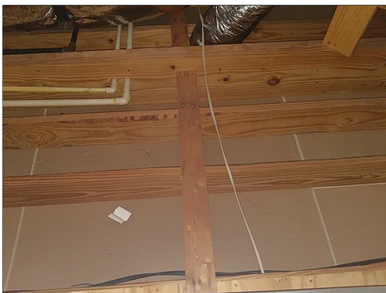
Upper attic area
